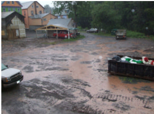
Disturbed area eroding during rainfall event
