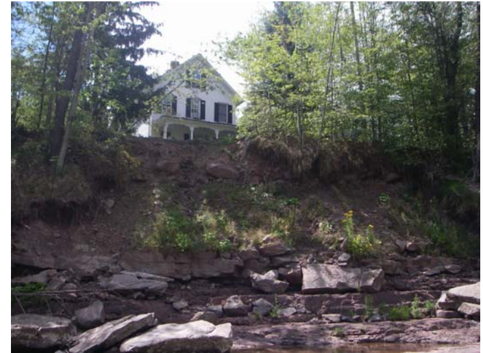
Left Bank, where VRSS would be installed
