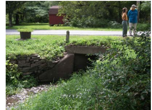
Culvert to be replaced
